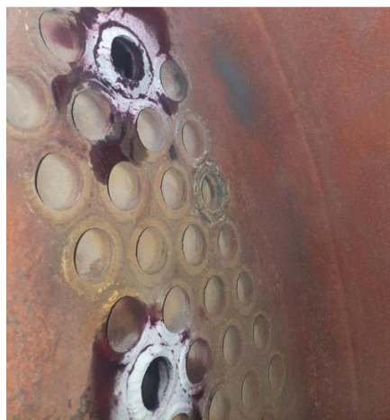
Figure 3. Front and back side of the boiler after repairs.
