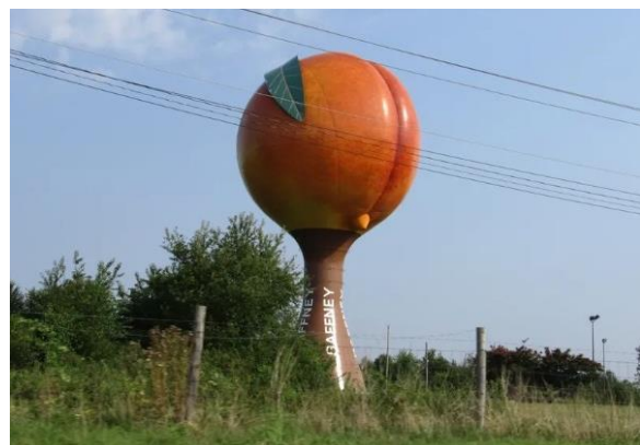
Figure 27. Peachoid water tower in South Carolina, /32/.
