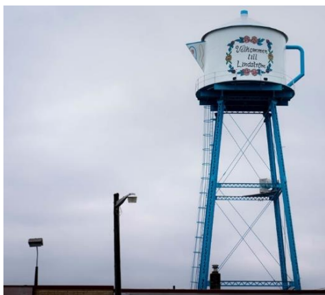
Figure 28. Swedish coffee pot water tower in USA, /33/.
