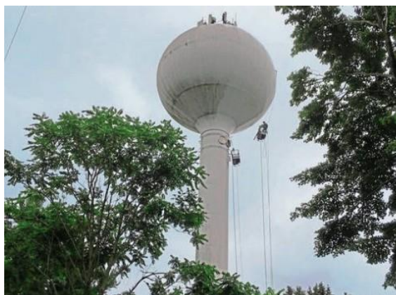
Figure 22. Spherical steel water tower during cleaning, /27/.
