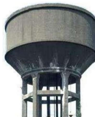
Figure 9. Intze water tower in service condition, /13/.
