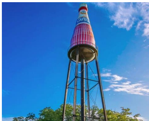
Figure 29. Bottle water tower in Collinsville, Illinois, /34/.
