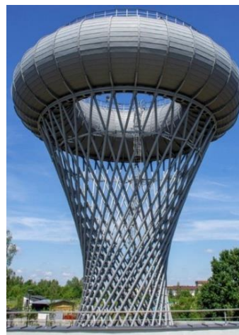
Figure 24. Toroidal steel water tower in Poland, /29/.
