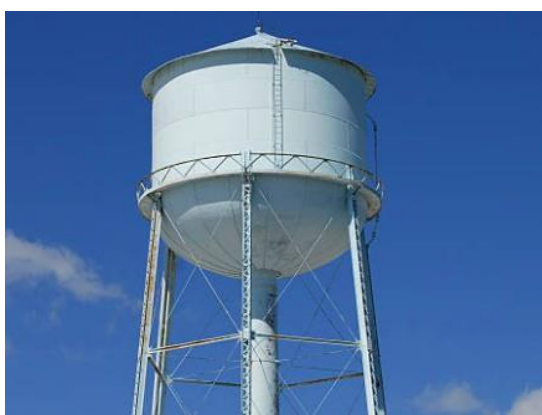
Figure 20. Cylindrical steel water tower with conical roof, /25/.
