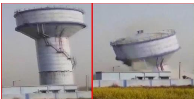
Figure A1. Collapse of a 700 m 3 reinforced concrete water tower due to poor-quality materials in Bankura, India, /43/.
