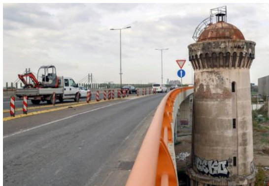
Figure 21. Spherical steel water tower, Gazela Bridge, /26/.
