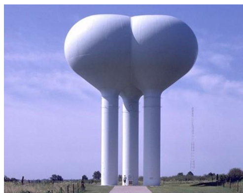
Figure 23. Polyspheroid water tower in San Diego, /28/.
