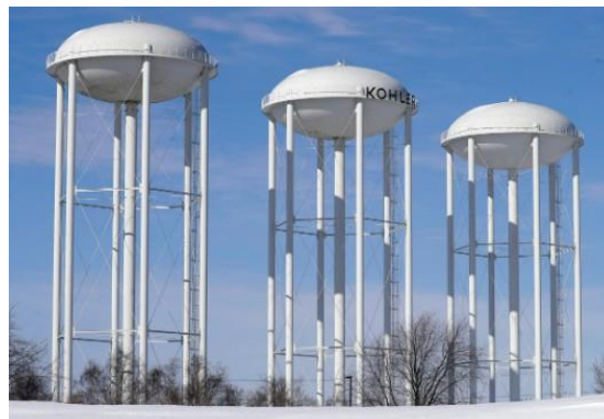
Figure 19. Kohler ellipsoidal water tower, Wisconsin, /24/.
