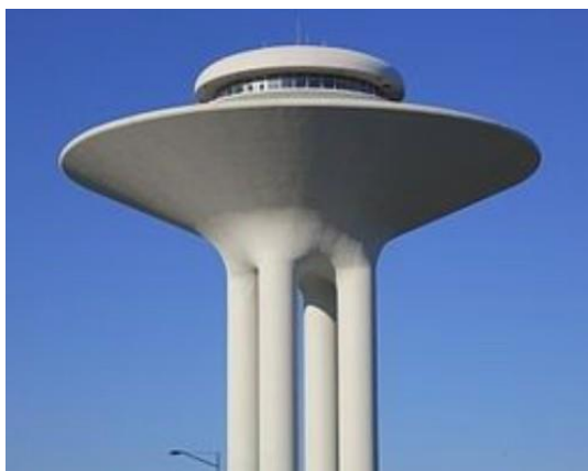
Figure 16. Hyllie water tower, Malmö, Sweden, /21/.
