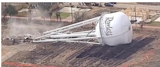
Figure A2. Collapse of a steel water tower due to a tornado in Texas, USA, in 2015, /44/.
