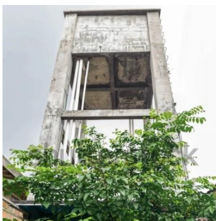
Figure 6. Rectangular reinforced concrete water tower, /12/.
