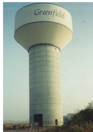
Figure 32. Composite water tower in service, /10/.
