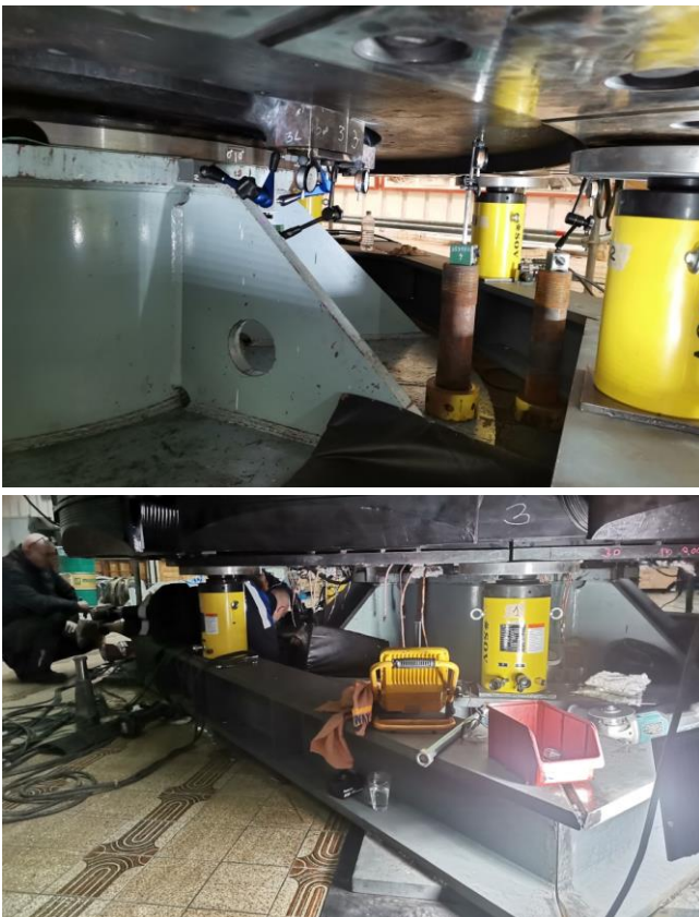
Figure 9. Hydraulic lifting and testing.
