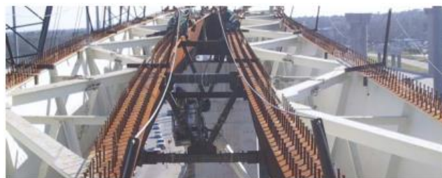
Figure 4. External connection system between box girders, /4, 5/.
