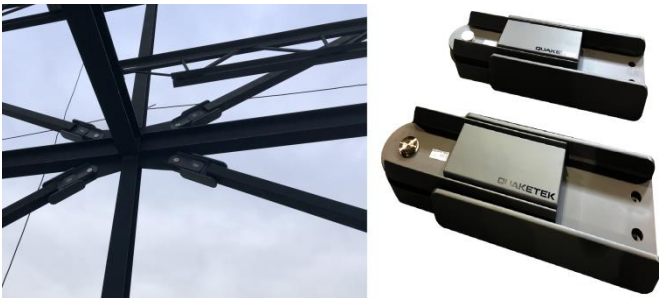
Figure 5. Friction damper application in steel farm structure.
