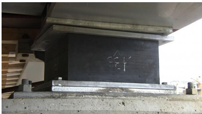
Figure 1. Lead-elastomer seismic isolator.
