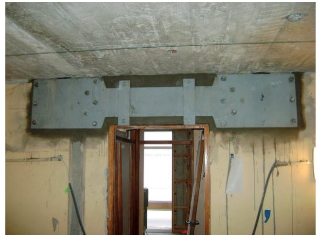
Figure 7. Viscoelastic damper application in a building.
