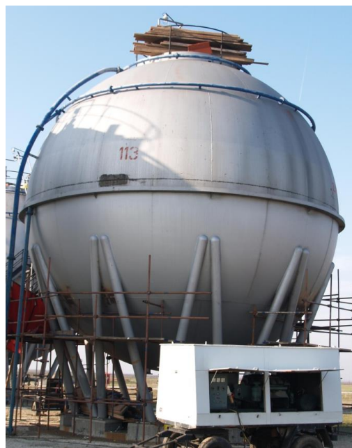
Figure 1. LPG spherical tank, designated as R-113.
