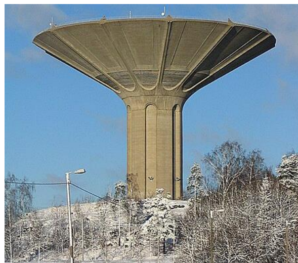
Figure 26. Concrete mushroom-shaped water tower, /28/.
