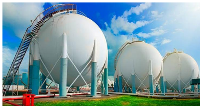
Figure 21. Horton sphere tanks, /22/.
