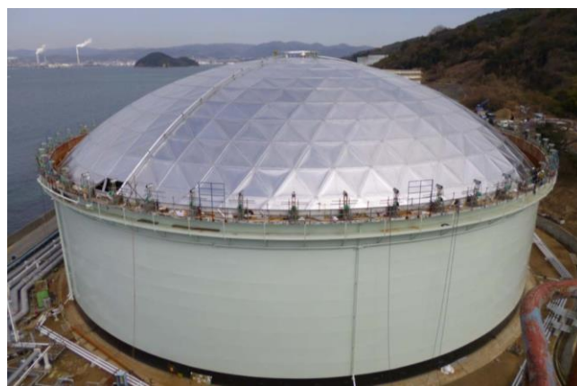
Figure 4. Geodesic dome roof tank, /11/.
