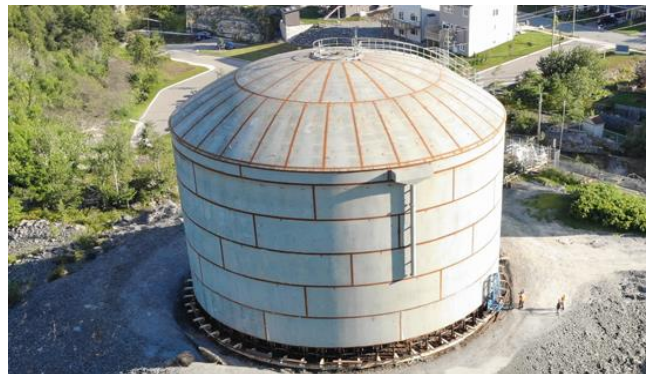
Figure 5. Tank with carbon steel dome roof, /12/.
