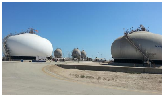
Figure 19. Segmented spheroid tanks, /18/.
