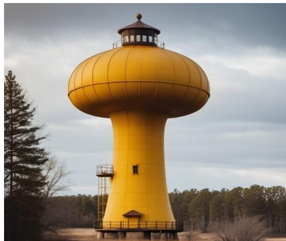
Figure 25. Carbon steel mushroom shaped water tower, /27/.
