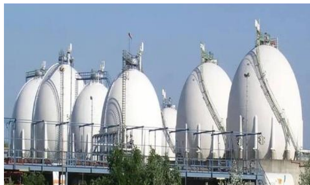
Figure 22. Elliptic tanks with a longer vertical axis, /23/.
