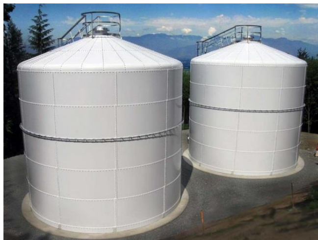
Figure 2. Storage tank cone roofs, /3/.
