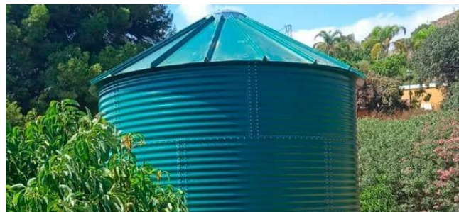
Figure 6. Tank with carbon steel self supporting roof, /12/.
