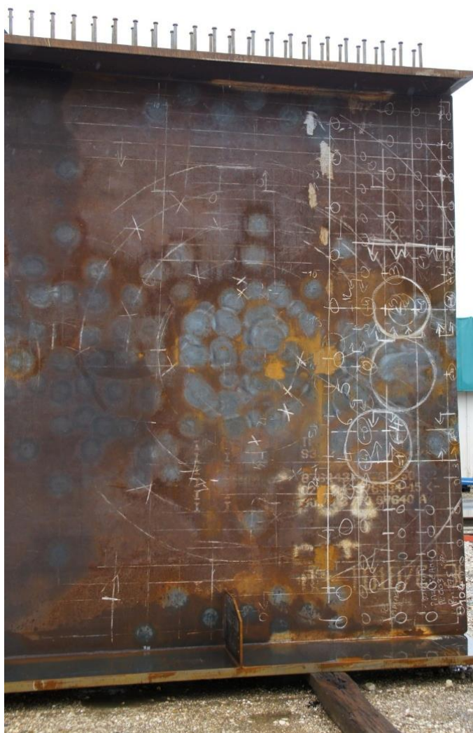
Figure 5. Image of the process used in France to correct a web with large deformations.
