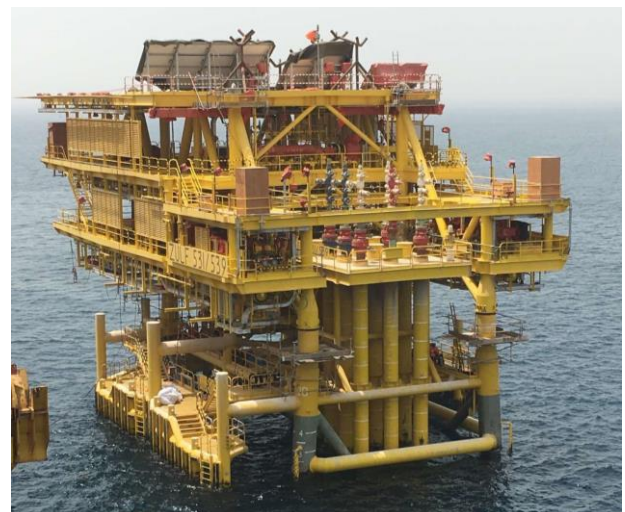
Figure 9. Offshore jacket after completed installation.
