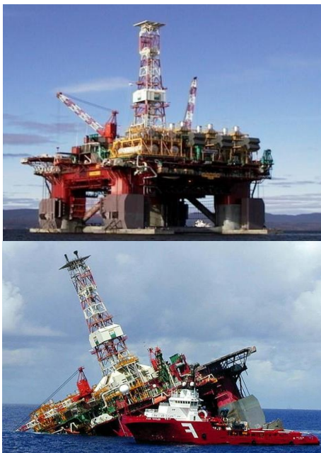
Figure 12. Petrobras-36 platform during work and sinking /24/
