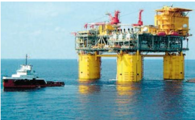
Figure 5 Magnolia oil platform in operation /11/
