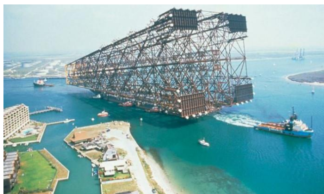
Figure 2 Transporting the Bullwinkle platform to the location /6/
