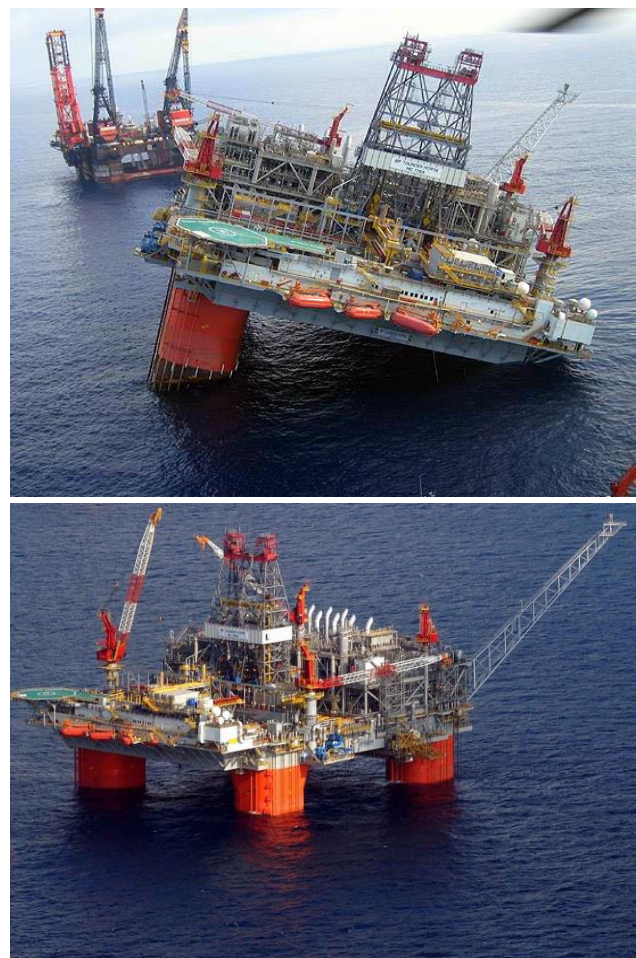
Figure 13. Thunder Horse processing platform after hurricane and after repair /25/
