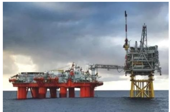
Figure 11. Balmoral platform-well production platform /24/
