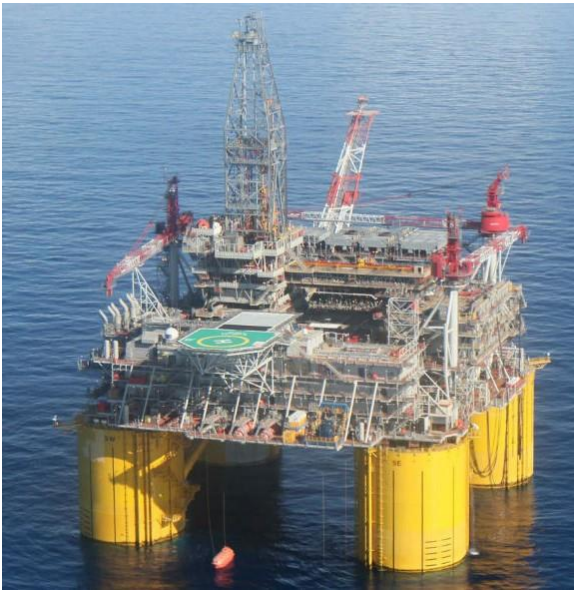
Figure 4 Olympus-Platform with tension legs /9/
