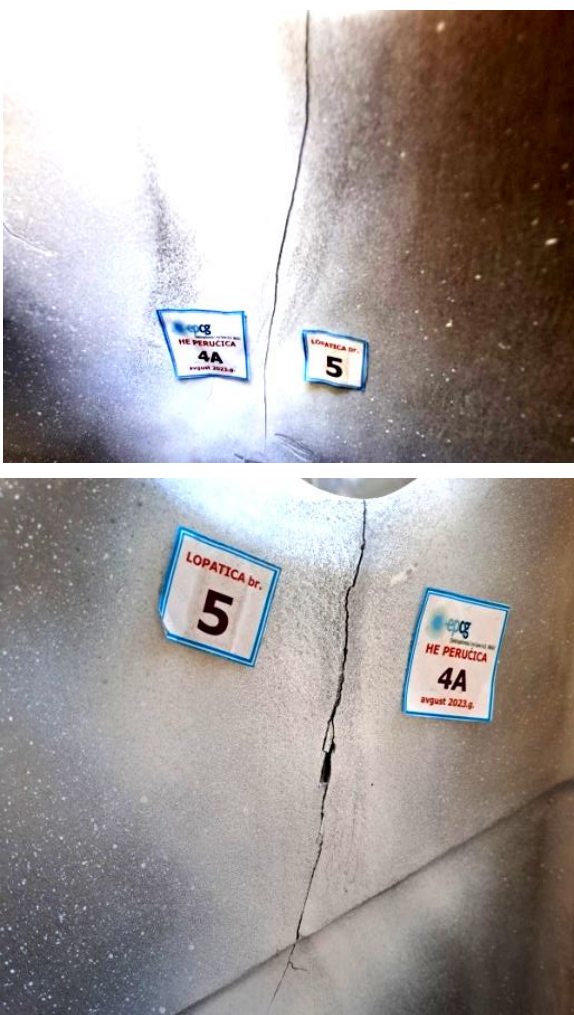
Figure 3. Detected crack on Pelton runner's blade length of 200 mm: top) front side; bottom) back side
