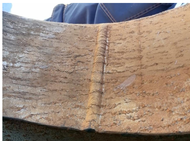
Figure 8. Caustic corrosion observed in the initial phase.
