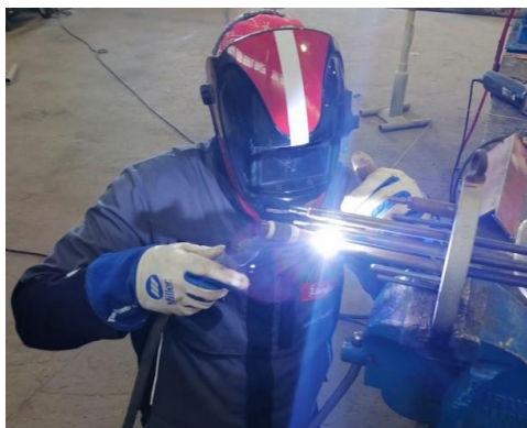
Figure 14. Repairing of the electric heater.
