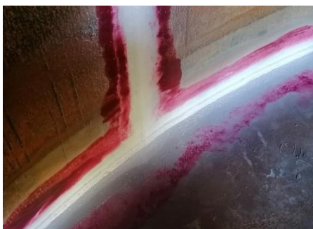
Figure 10. T-welded joint after developer spraying (no cracks).
