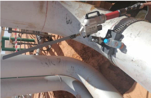
Figure 8. Cutting of a damaged elbow in a safety manner.
