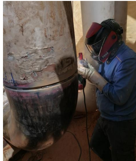
Figure 9. Welding of the new elbow to the manifold line.
