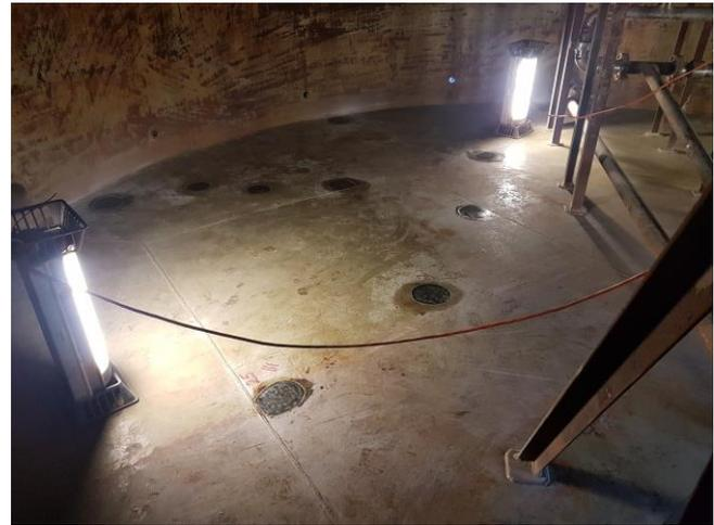
Figure 8. Thickness measuring points according to created random ultrasonic schemes.
