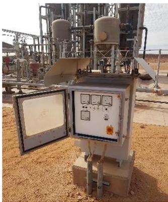
Figure 9. Cathodic protection cabinet after opening and current stimulation from control room.
