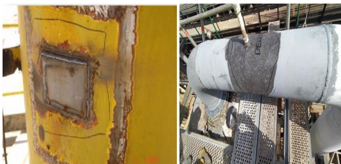
Figure 2. Reparation of the corroded area.
