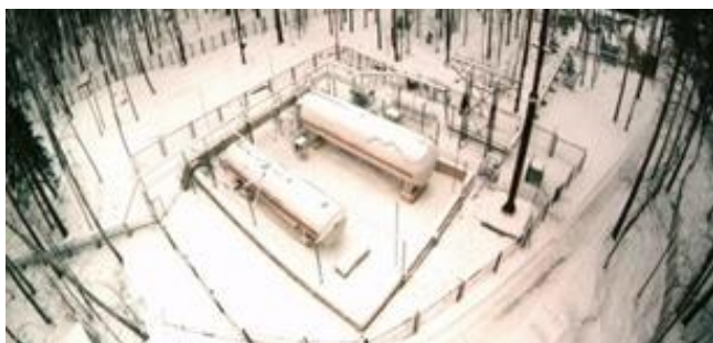
Figure 5. Cryogenic tanks, 40 m 3 , for LNG storage and regasification for subsequent gas supply boiler room.
