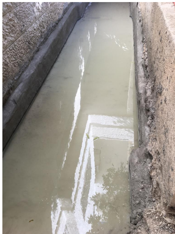
Figure 11. Seepage testing technique.
