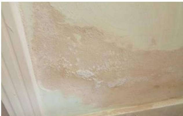
Figure 4. Damp on different locations of the internal walls.
