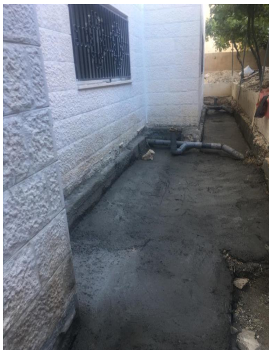
Figure 8. Casting of concrete before flooring.
