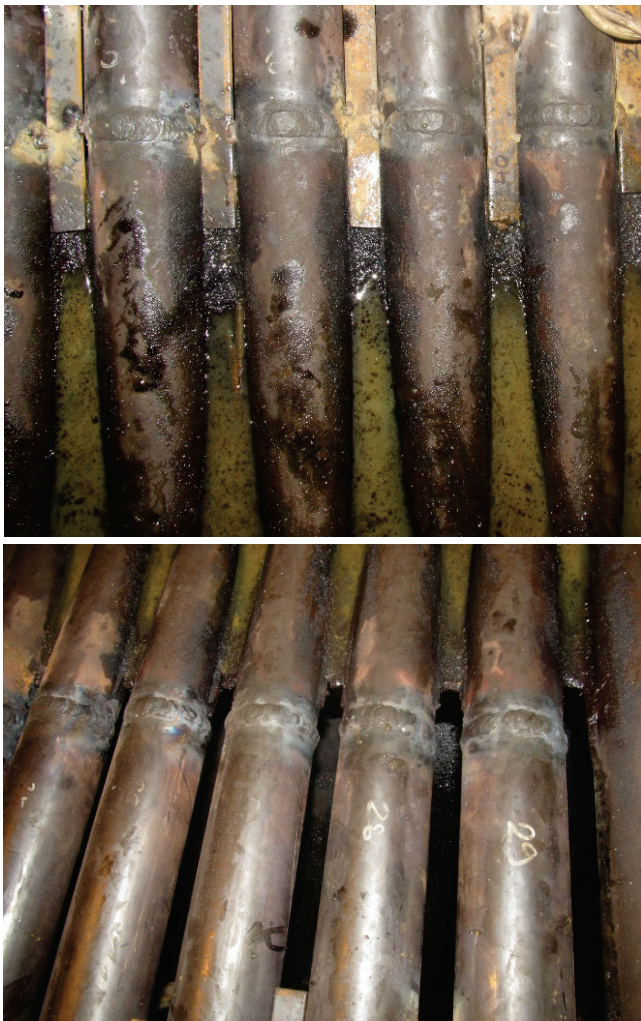
Figure 7. Joining new and old tubes of the bottom panel.
