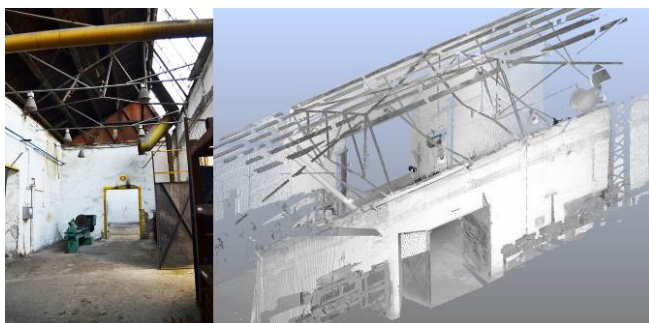
Figure 6. Photograph and 3D scan of bended trusses.
