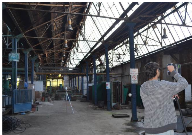
Figure 2. Scanning of the workshop interior.
