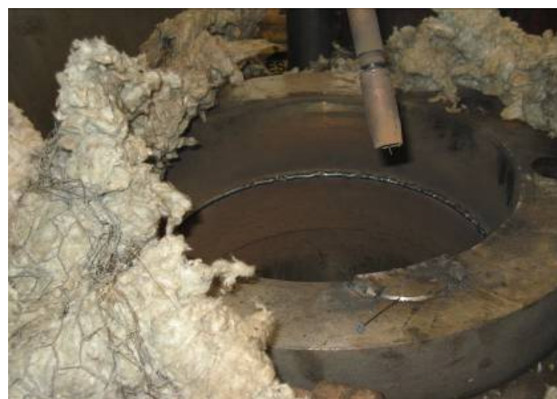
Figure 3. Device ID Weld 2501 for surface welding performed at the openings of guide vane cranks.
