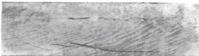
Figure 1. Cracks at the shell-head welded joint of the storage tank. Slika 1. Prslina u zavarenom spoju omotača-danca rezervoara
