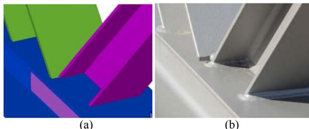
Figure 6. Truss beam joint (a) designed (b) manufactured – imperfection type 2.
