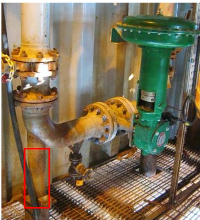
Figure 4. Support failure.
