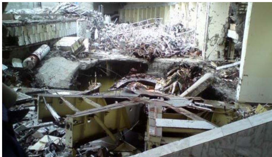
Figure 1. Scene of the Sayano-Shushenskaya hydroelectric power station after the accident, /1/.
