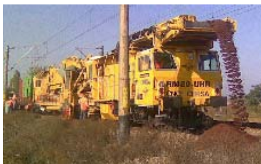
Figure 2. Ballast cleaning machine.
