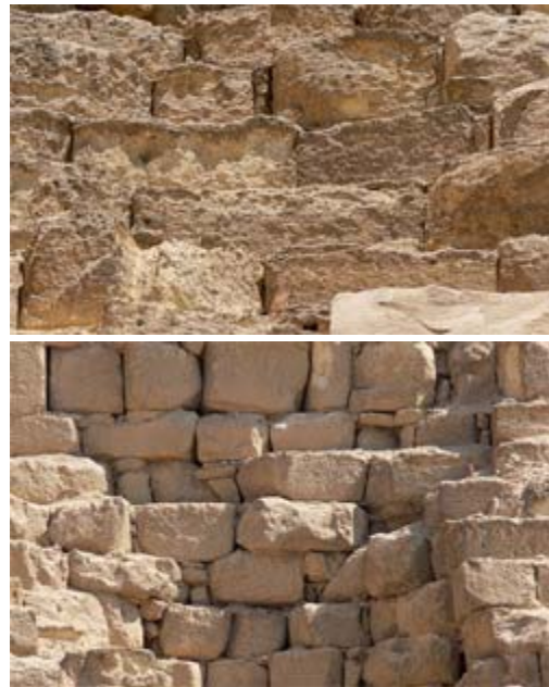
Figure 3. Blocks that appear to have been cast (top); blocks most likely not cast (bottom).
