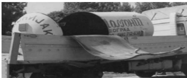
Figure 14. Plastic collapse of transportable storage tank (II), /21/ Slika 14. Plastični lom transportne cisterne (II), /21/
