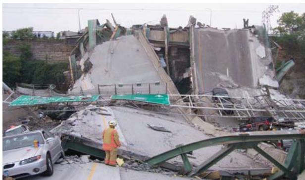
Figure 7b. The collapsed bridge, 1 st August 2007, /10/ Slika 7b. Srušen most, 1. avgusta 2007, /10/
