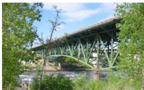
Figure 7a. The bridge before the collapse, /10/. Slika 7a. Most pre kolapsa, /10/
