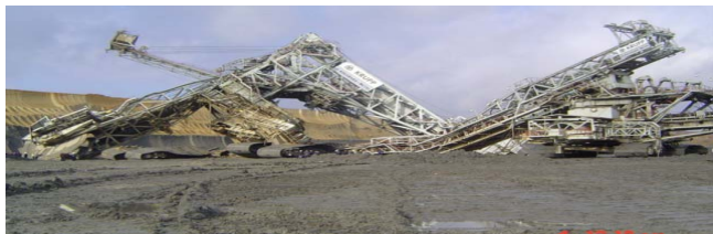
Figure 15. Collapse of bucket wheel excavator, /1/. Slika 15. Kolaps rotacionog bagera, /1/
