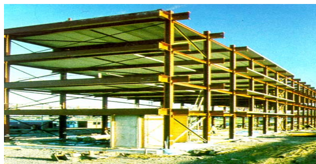
Figure 1. High-rise parking building (under construction). Slika 1. Višespratno parkiralište (u izgradnji)
