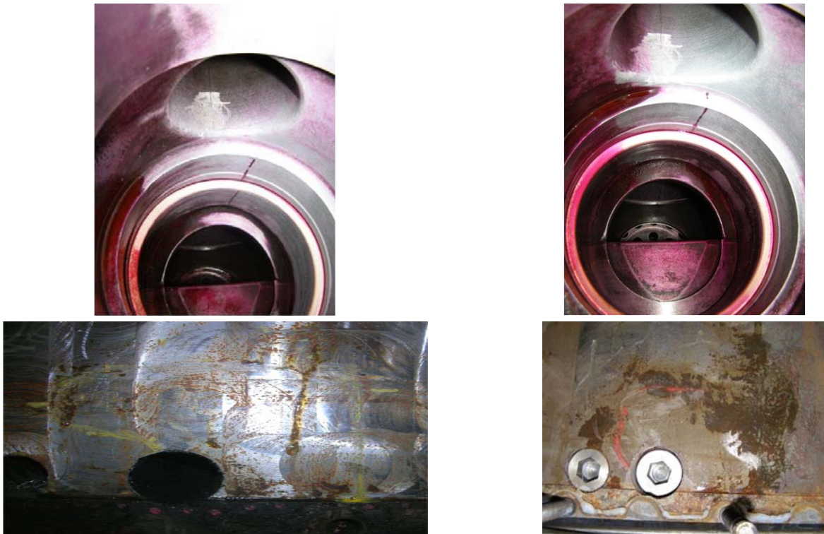
After 15 days operation, inspection has validated the calculations and the applied data, checking crack size and position.
