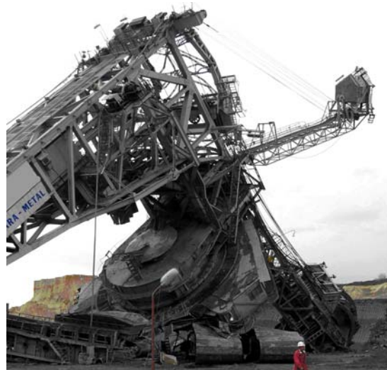
Figure 16. Collapse of rotor excavator. Slika 16. Kolaps rotornog bagera
